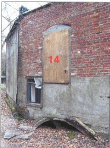
North side of Building 14 (Dye House, after 1922).
