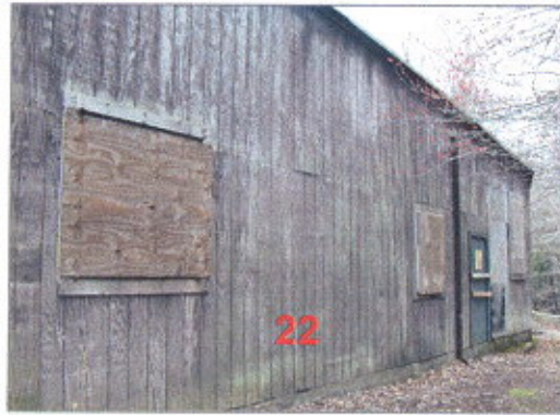
Northeast corner of the mill complex.
