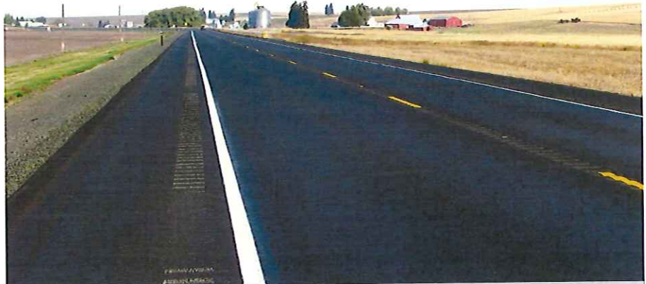
Shoulder rumble strips and center line rumble strips are installed on this roadway.
