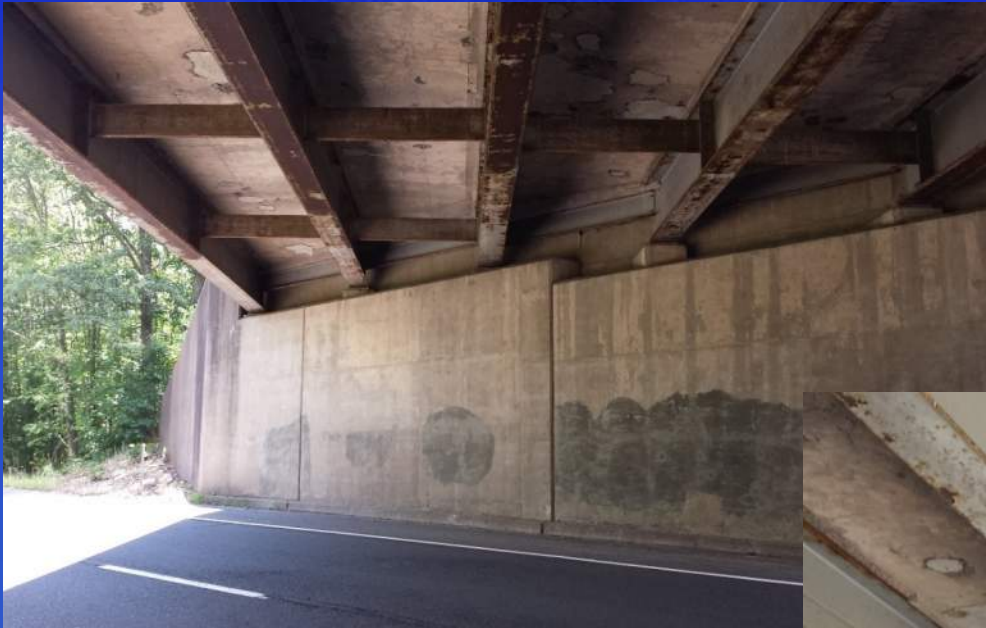
Underside of Bridge and West Abutment
