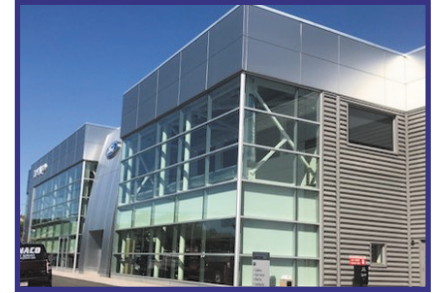
Newly completed Monaco Ford facade.
