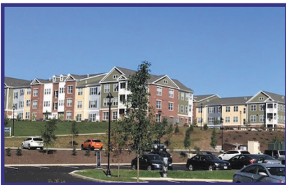
The Tannery Redevelopment Project
