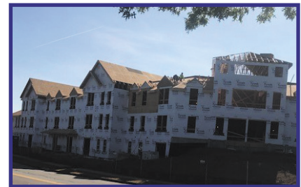
Center Village (in construction)
