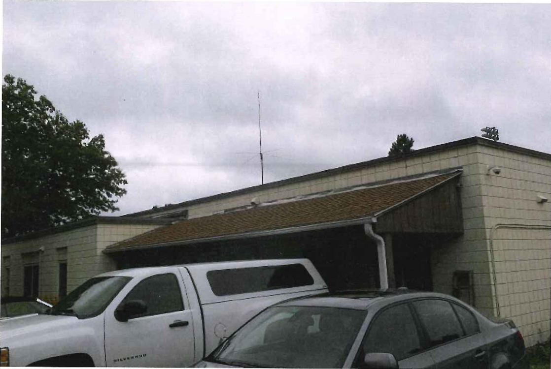
Front entrance and covered porch area
