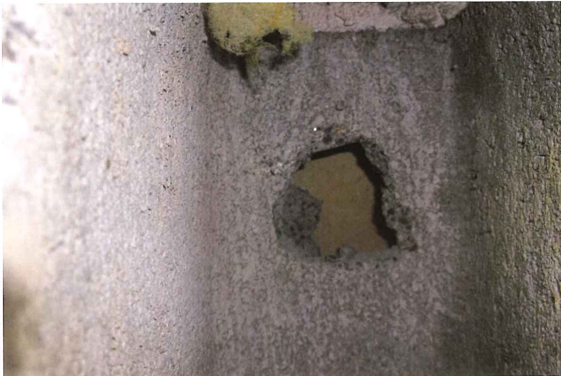
Interior cavity exterior CMU block
