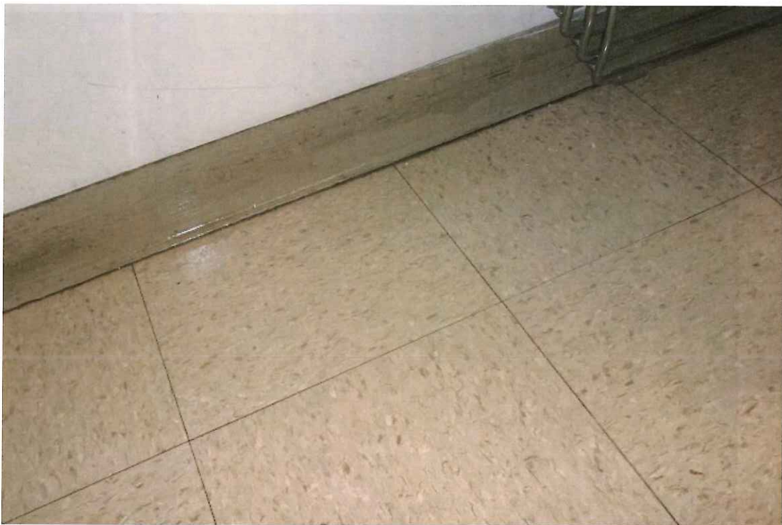
Floor tile and cove base break room
