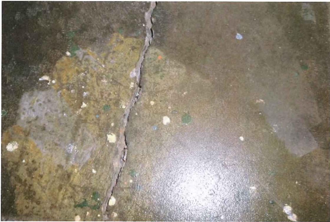
Carpet adhesive storage room #1
