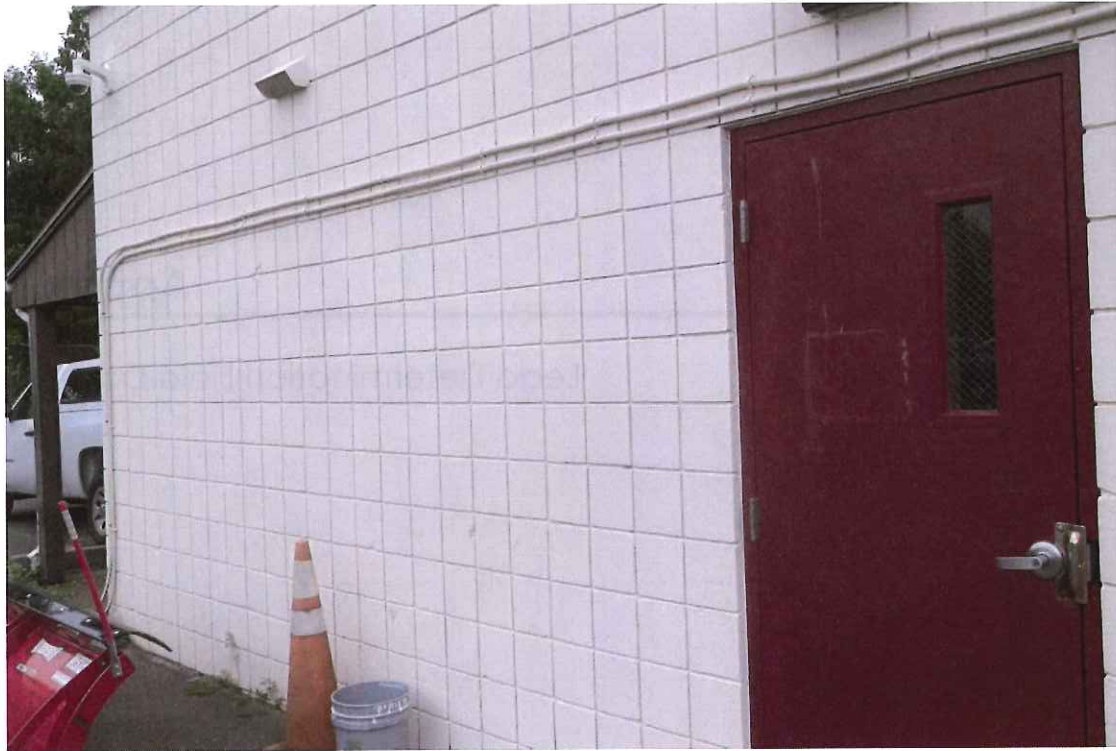
Exterior CMU block
