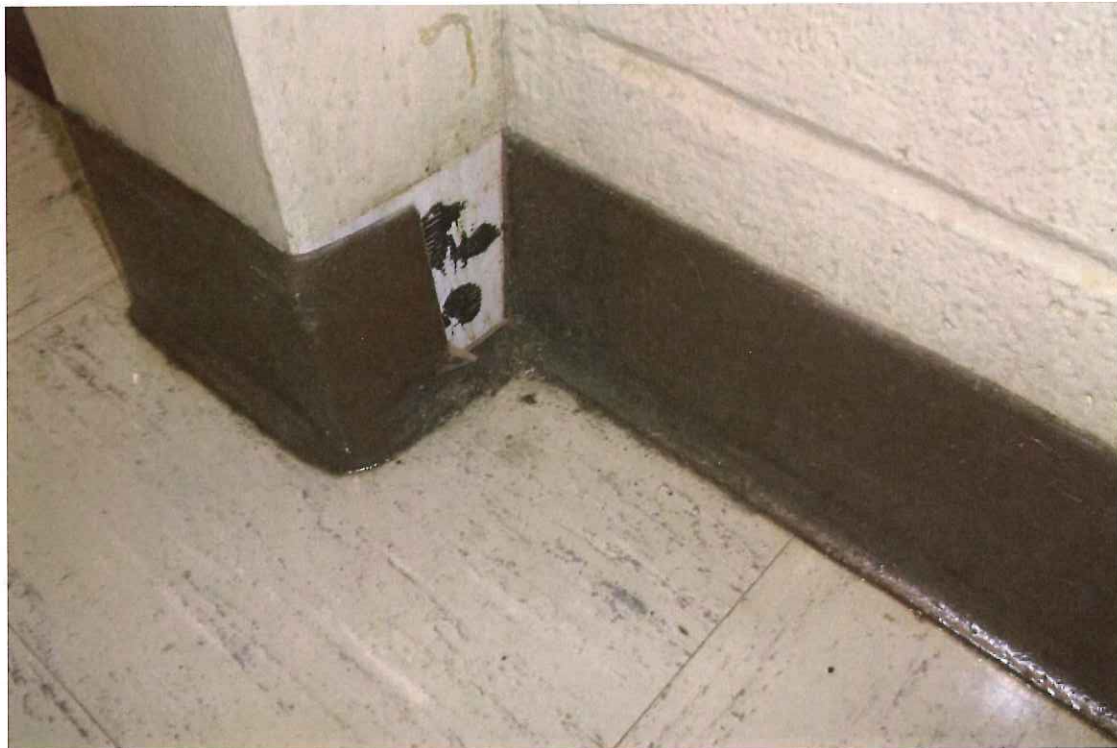
Bathroom #1 floor tile and cove base
