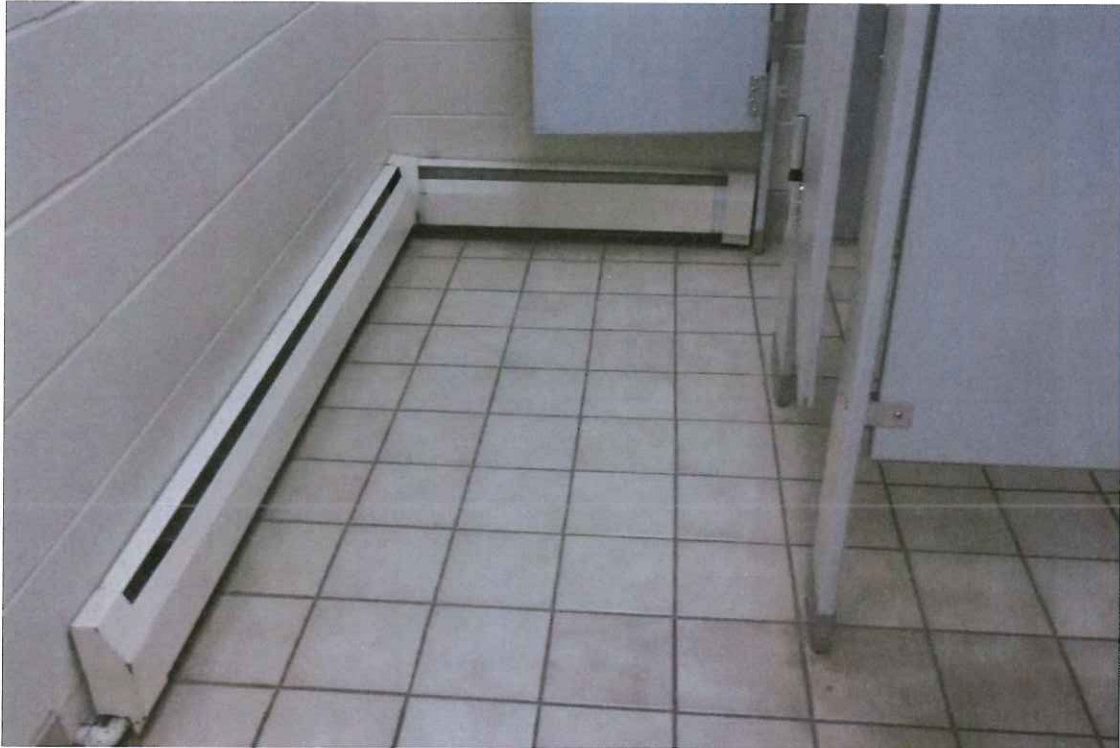
Ceramic floor Bathroom # 2 shop area
