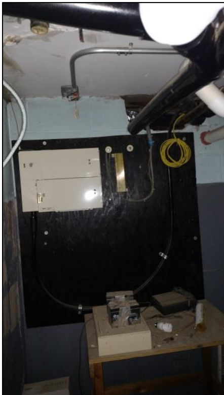
25 Risley Road (Basement)
