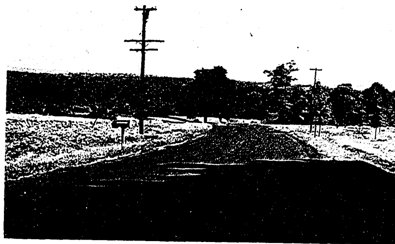
Route 94, or Hebron Avenue, was originally a State Aid road and is now a part of the Connecticut State highway system. The view shows the road looking west from John Tom Hill.
