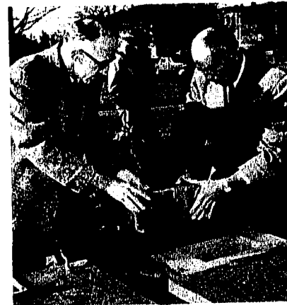
Mr. Martin Roser, Chairman of Public Building Committee, and Mr. Sayre B. Ross, former Chairman of the Town Council, laying corner stone for new Town Office Building.
