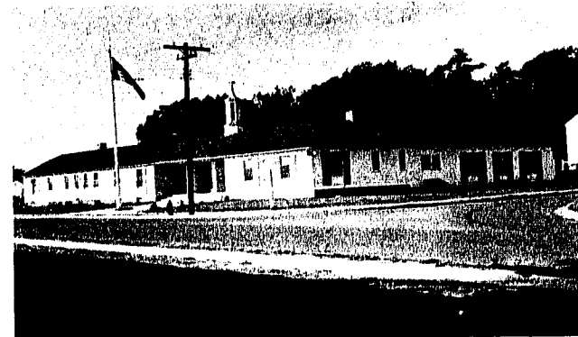
ADMINISTRATION BUILDING AND COMMUNITY HALL IN WELLES VILLAGE
