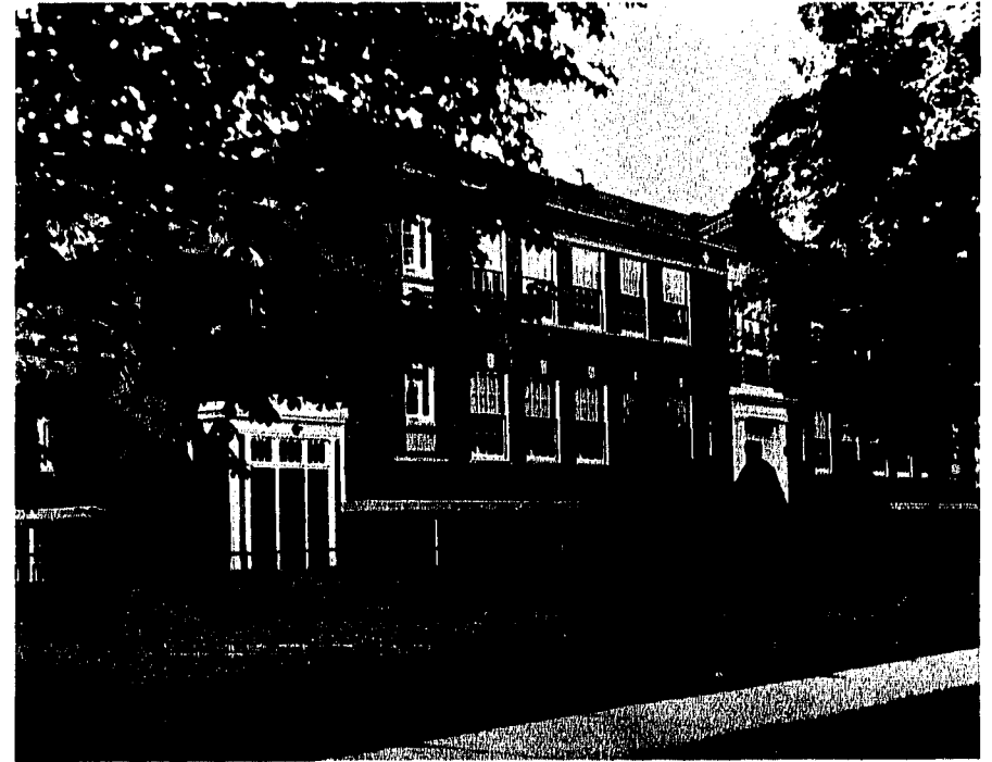
ACADEMY SCHOOL. This school will be converted to a Junior High School.
