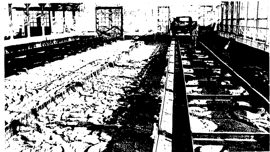
Sludge-drying beds at Treatment Plant.
