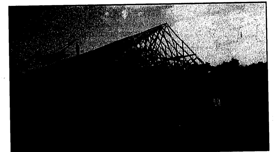
Construction at Company 3 Firehouse.
