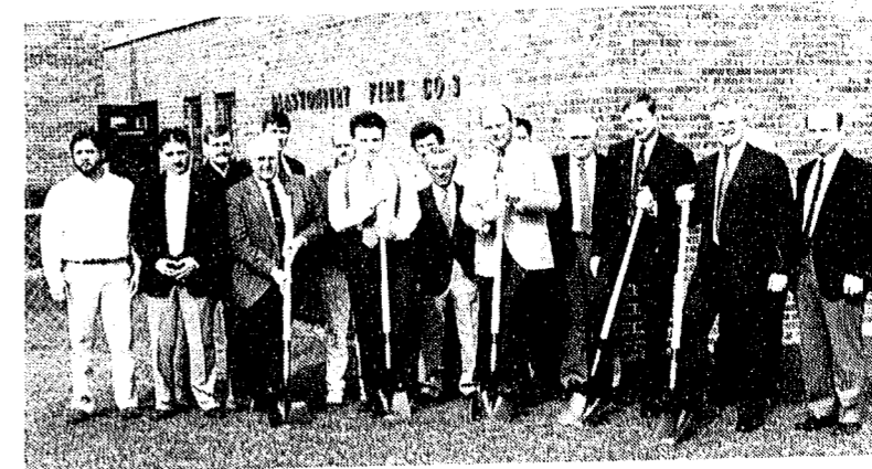
The traditional ground-breaking ceremony for the renovations to Fire Companies #3 and #4. Shown above with shovels are (left to right), Fire Chief Mario Accornero, Town Council Member Paul Nye, Fire Commission Chairman Gil Spencer, Town Manager Richard Borden and Public Building Commission Chairman David Megaw.
