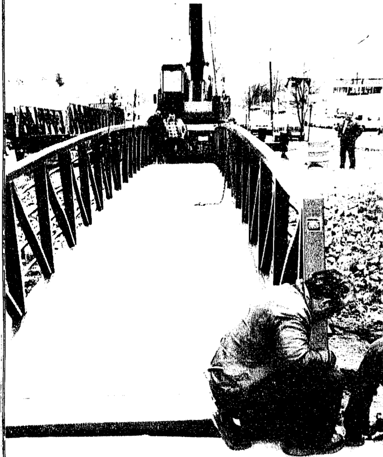
A footbridge was installed over the brook just east of the Bemer/Volkswagon complex to allow pedestrians to reach the shopping center. The preconstructed bridge was lowered by crane on to readied foundations in a matter of minutes, an exercise in trained precision.
