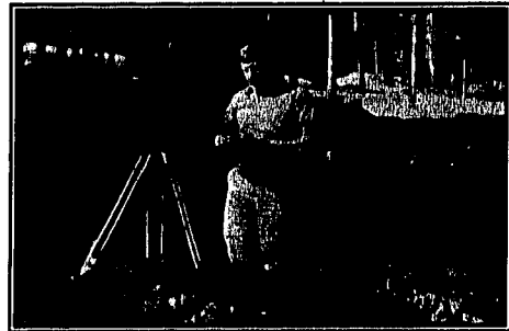
Sanitarian David Brunelle conducts final site inspection for residential on-site sewage disposal system.
