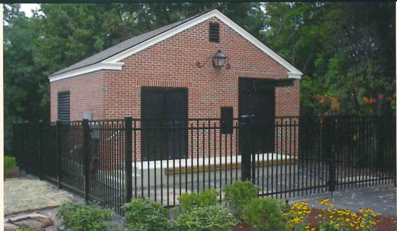
Pump Station located at the corner of Main and Hubbard Street.
