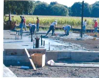
Contractors place concrete foundations at the new Riverfront Community Center.
