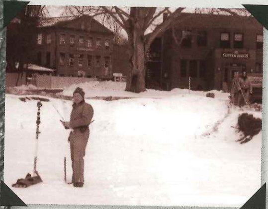
Engineering Division employees Rob Edwards and Doug Whitton provide grade elevations for the "new" Welles Street.
