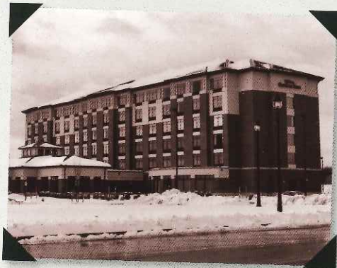
The new Hilton Garden Inn on Glastonbury Boulevard.
