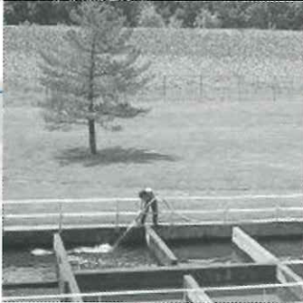
Cleaning the chlorine contact chambers at the Water Pollution Control Facility.
