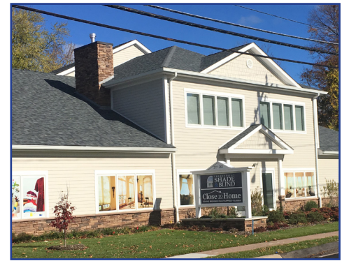
Pictured from top to bottom: 2520 Main Street, home to Firehouse Subs and Pet Valu; the Tannery building; First & Last Tavern; and CT Shade and Blinds.
