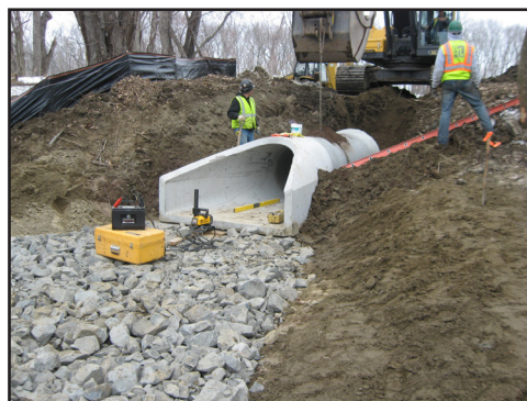
Setting new pipe outlet at CT River.
