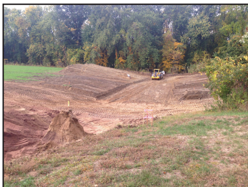
Initial excavation work.
