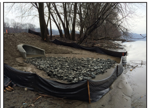
Completed pipe outlet at Connecticut River.
