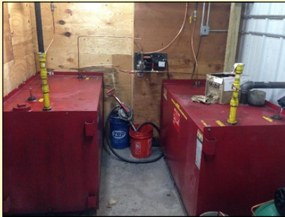
Holding tanks used to store waste oils connected to fuel troth.
