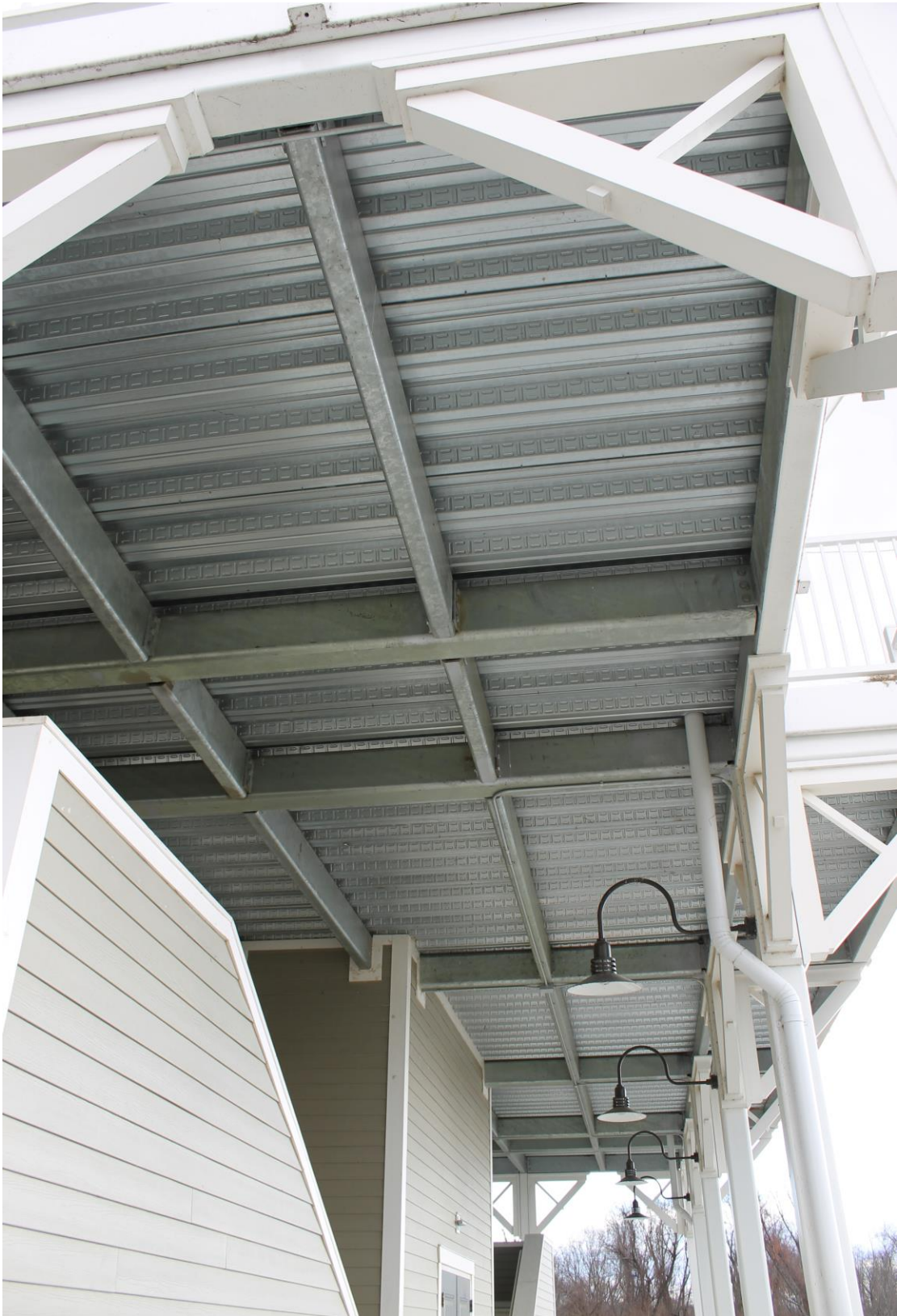
Underside of deck above first floor patio
