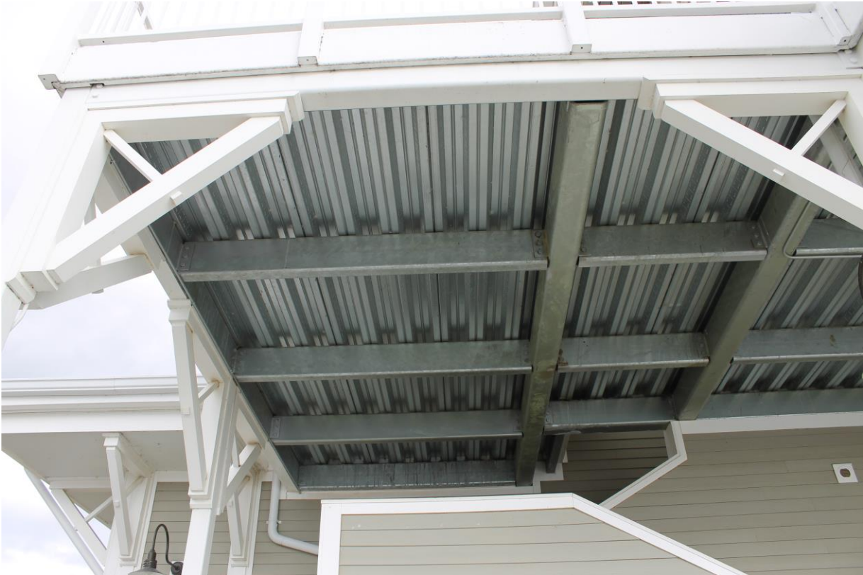
Underside of deck above first floor patio
