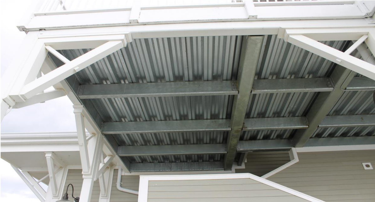
Underside of deck above first floor patio
