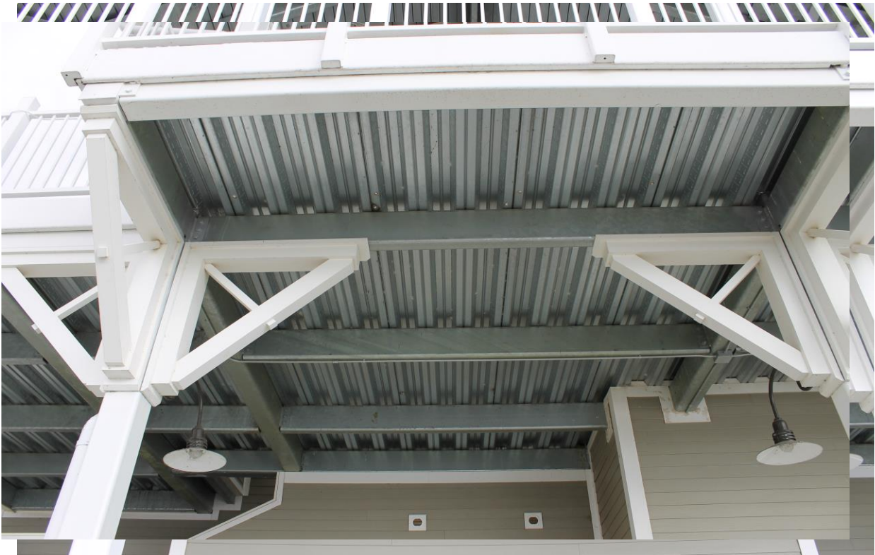
Underside of deck above first floor patio
