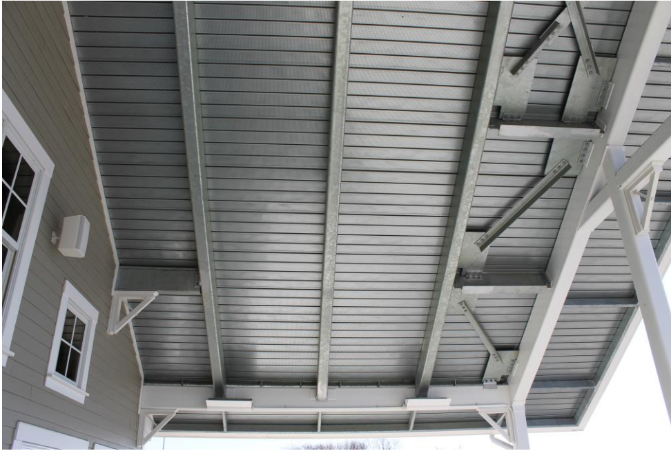
Underside of covered deck roof on second level
