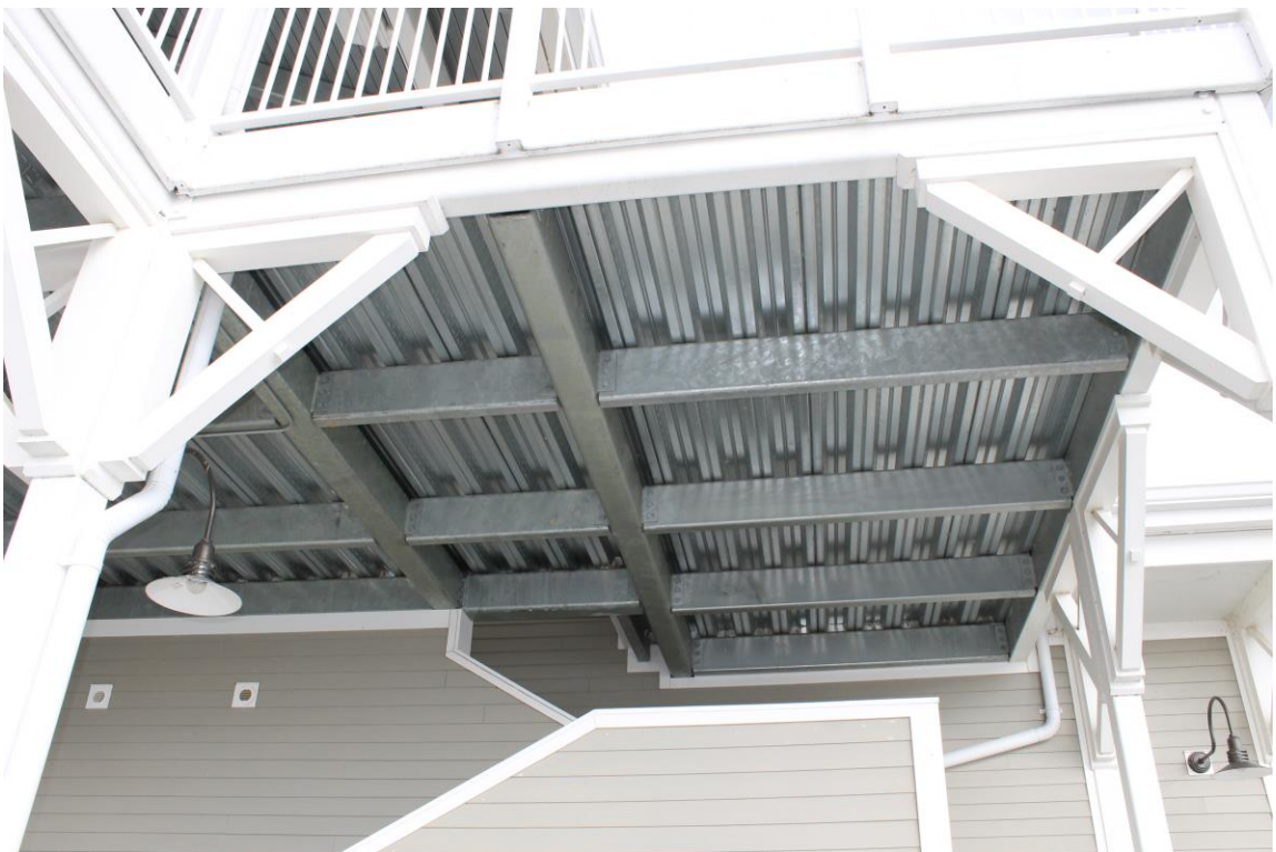
Underside of deck above first floor patio
