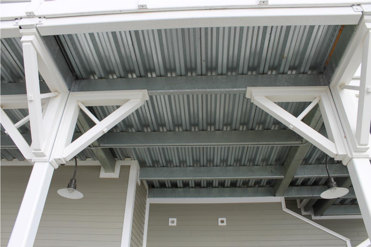
Underside of deck above first floor patio
