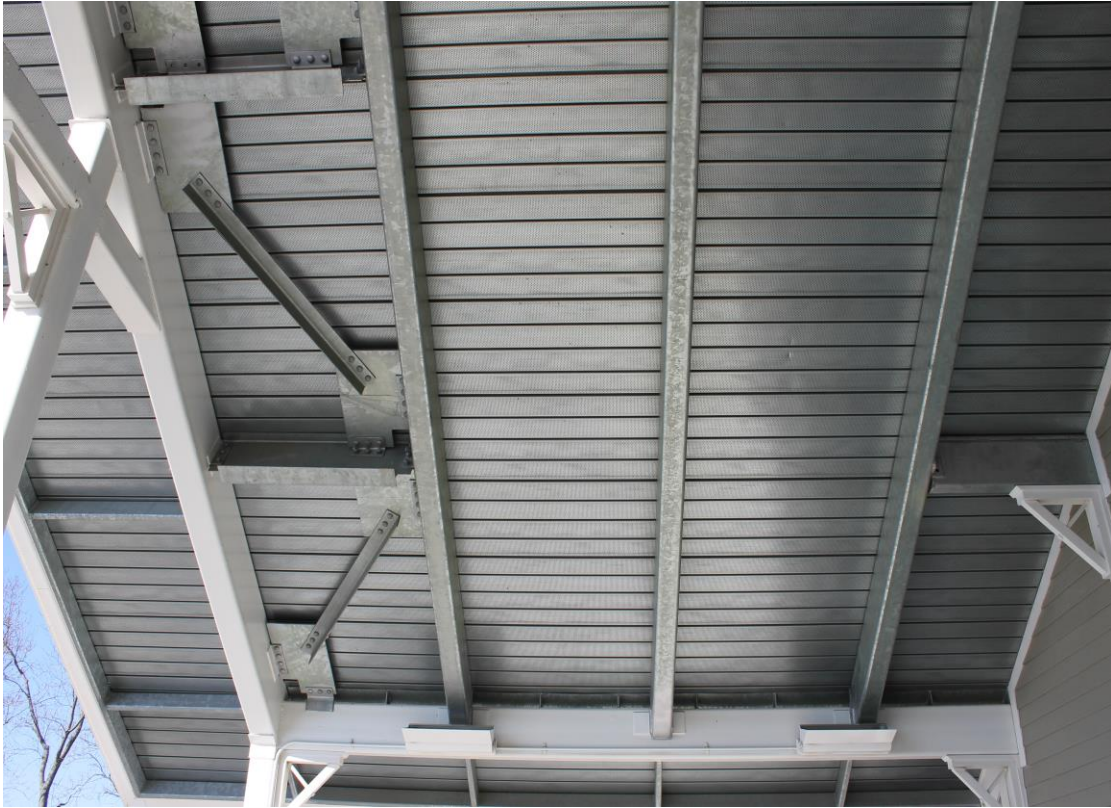
Underside of covered deck roof on second level
