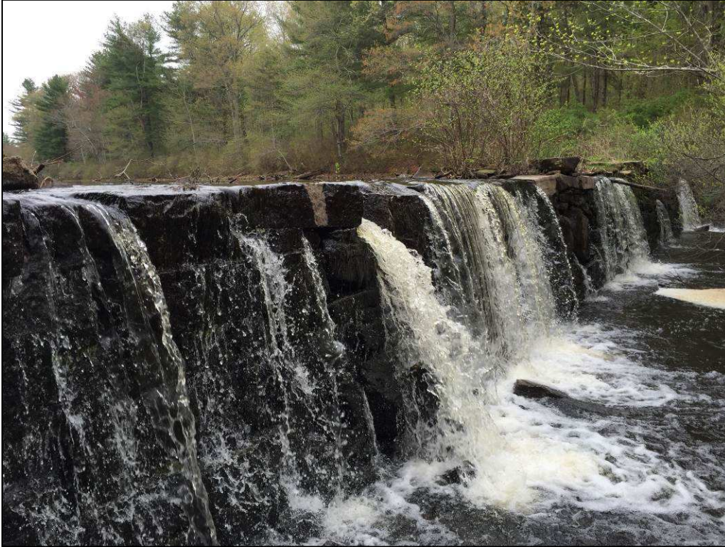
Photo 1: dam looking east.
