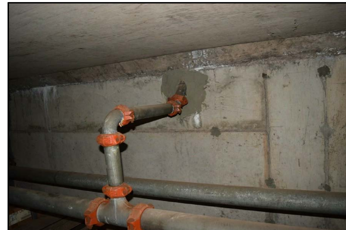
TYPICAL EXISTING GUTTER DRAIN PIPING
