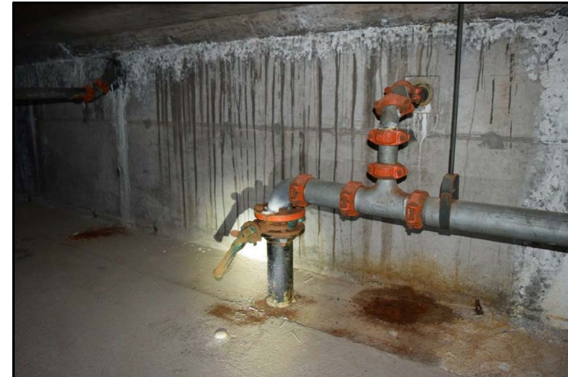
TYPICAL EXISTING GUTTER DRAIN PIPING
