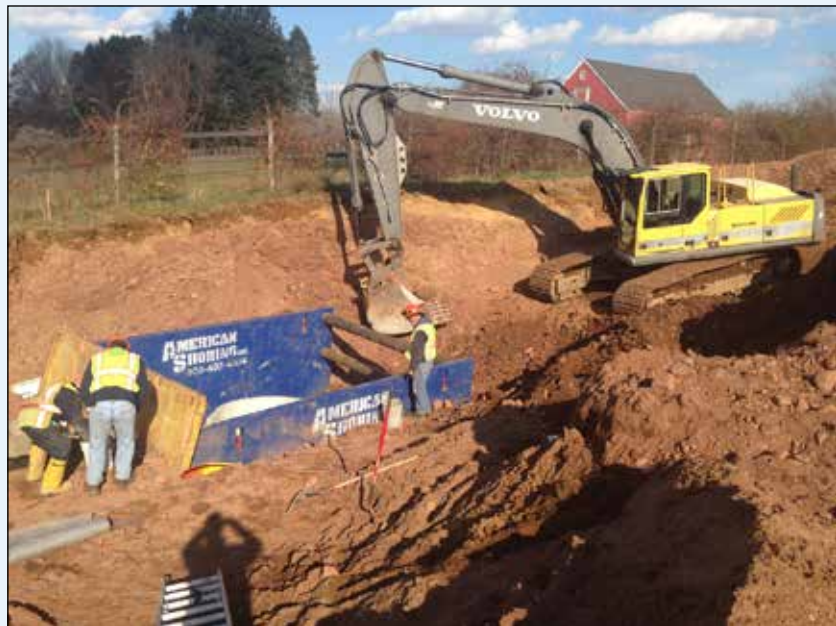
Highway Division staff working on the Tryon Street Drainage Project
