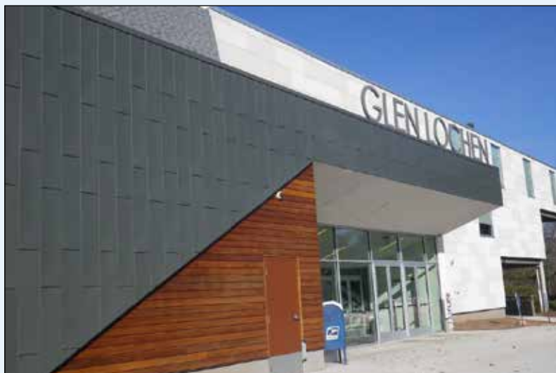
Newly renovated Glen Lochen Commercial Building on New London Turnpike
