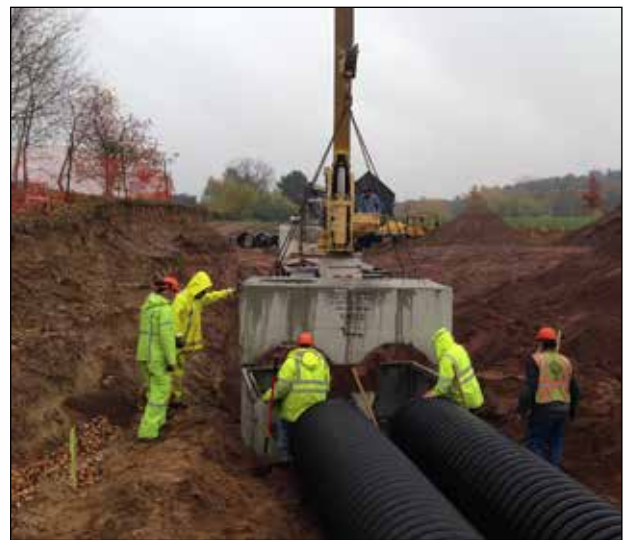
Highway division crew installing a drainage structure
