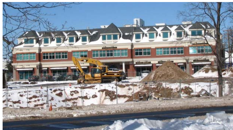
Eric Town Square under construction.
