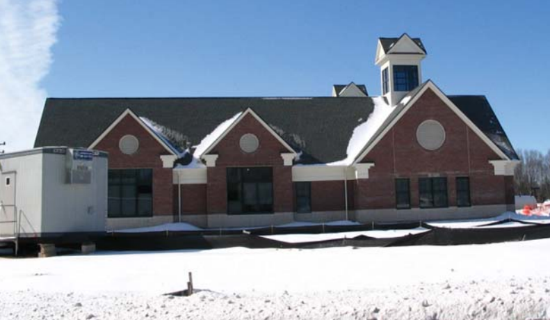
Eastern Boulevard under construction.
