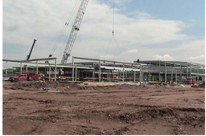
New elementary school steel erection.
