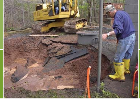
Water Pollution Control construction site
