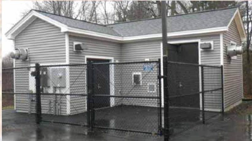
Nutmeg Pump Station upgrade
