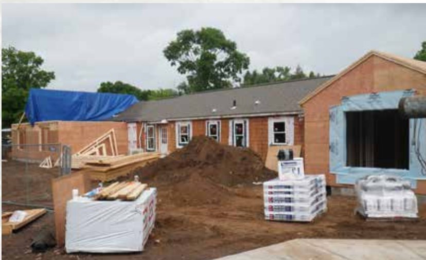
One of the buildings under construction at The Village Green
