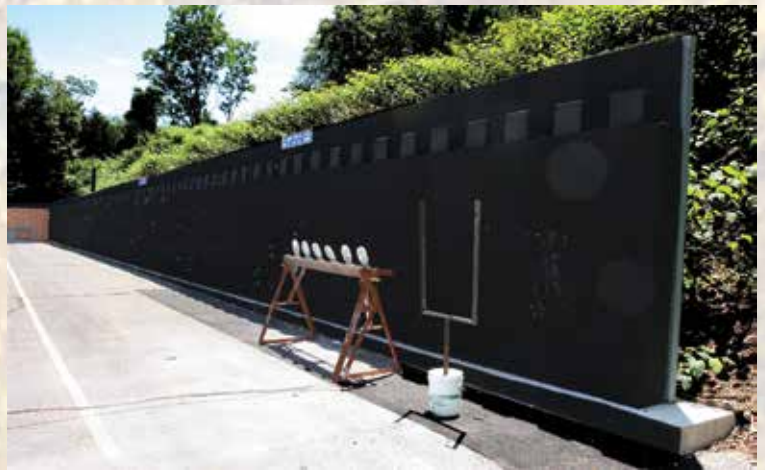
The new ecologically-friendly bullet trap at the fire arms range
