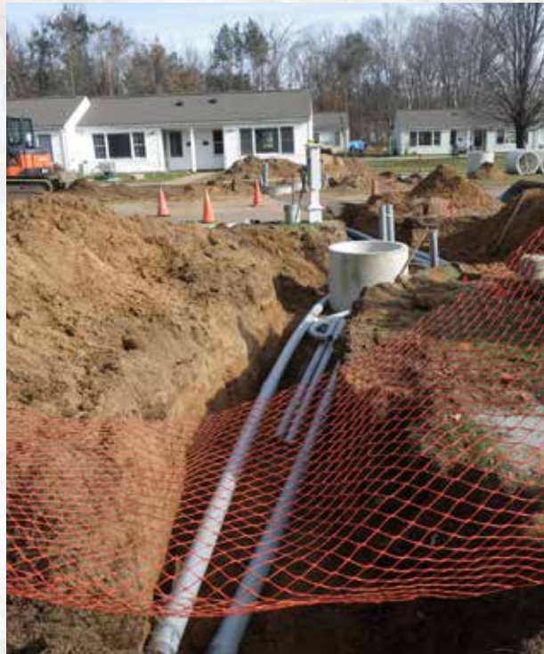
Site work and the property before building renovations started
