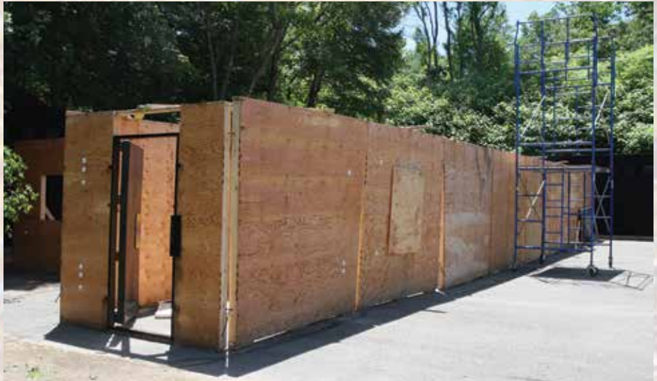
Newly constructed shoot house that allows for live fire training inside a simulated house. It can be reconfigured to change the floor plan
