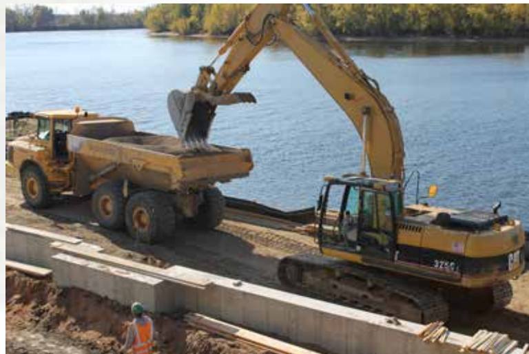
Work on the Riverfront
