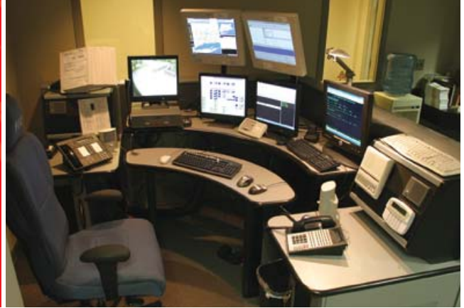
The Glastonbury Police Department's fully modernized communications center.
